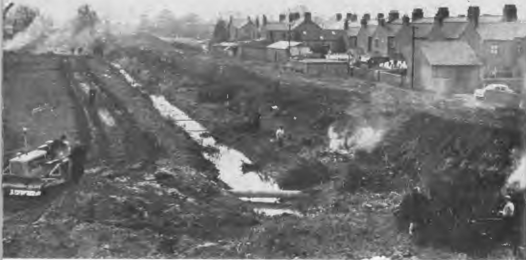
The route of the new by-pass takes shape. The embankment in which the Board's cables were buried formerly ran along the right of the picture.
