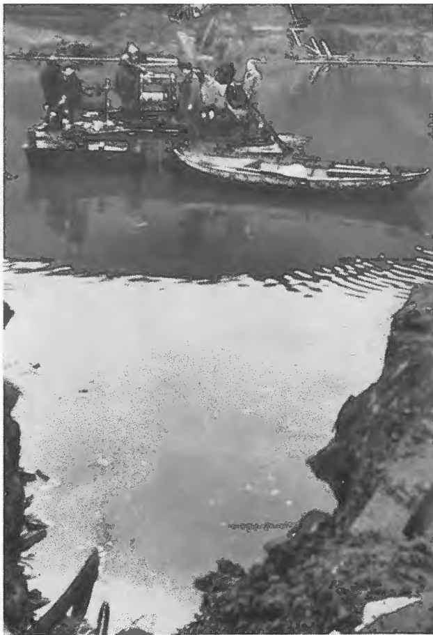
Hauling the cable across by barge.
